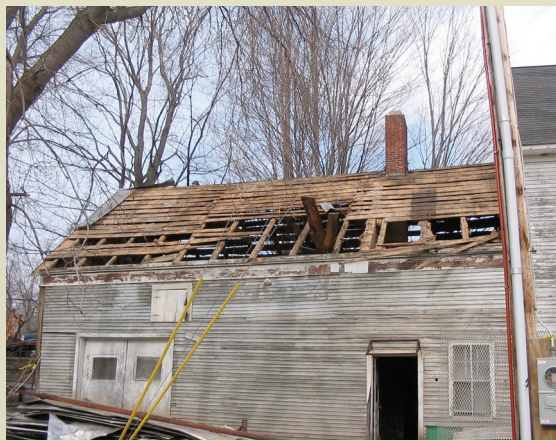
Deconstruction and salvage operation by Recycle North and Conner and Buck Builders. $12,000 worth of building materials were reclaimed and recycled back into the community.
