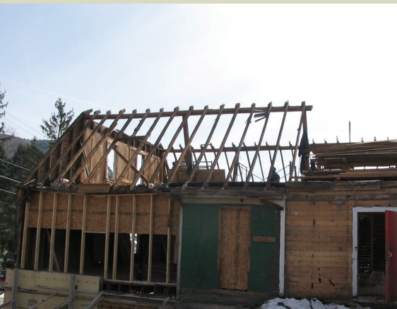
Deconstruction and salvage operation by Recycle North and Conner and Buck Builders. $12,000 worth of building materials were reclaimed and recycled back into the community.
