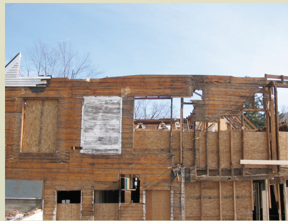
Deconstruction and salvage operation by Recycle North and Conner and Buck Builders. $12,000 worth of building materials were reclaimed and recycled back into the community.
