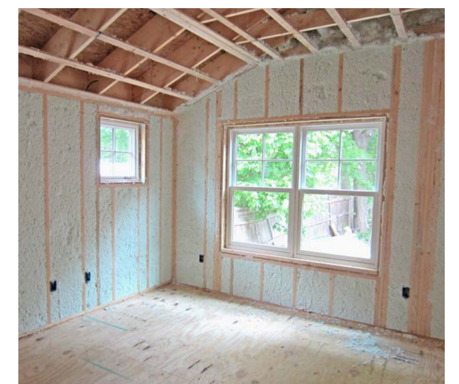
Spray fiberglass insulation at the new addition.
