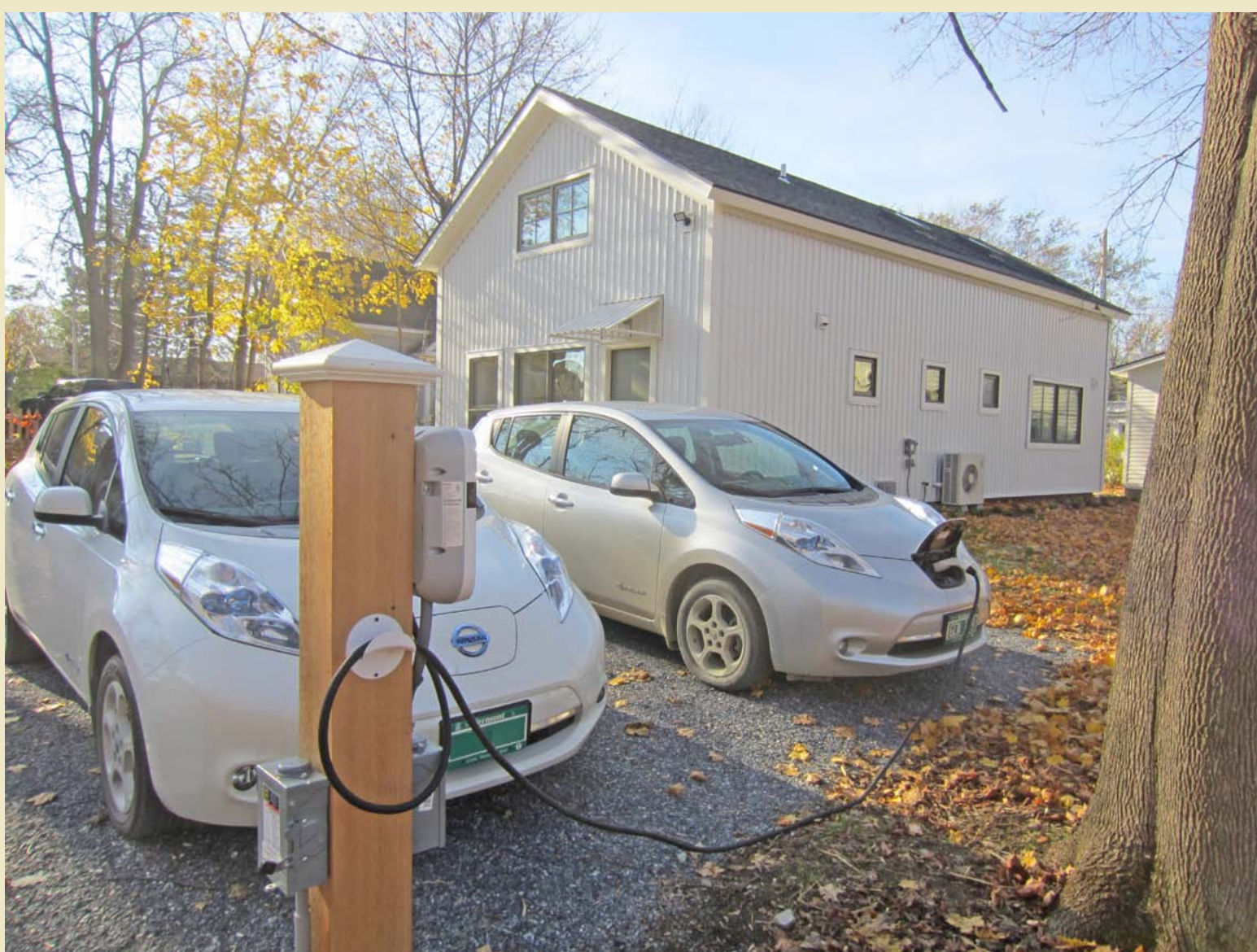
Electric vehicle charging
