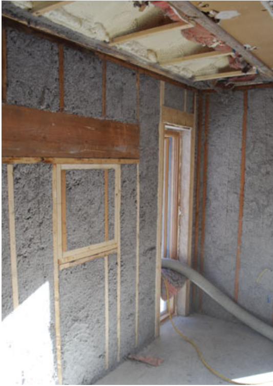
Figure 6. Spray-foam was used to seal the plates and boost R-values at the truss heels, and any open stud bays were filled with damp-spray cellulose (left). After the sheathing was wrapped with housewrap, window and siding installation was typical (above).
