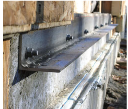
Figure 5. Sections of 3\frac{1}{4} -inch by 3\frac{1}{4} -inch by \frac{1}{4} -inch steel angle were bolted to the wall underneath the door openings (left and above). The angles were then padded with PT blocks and shims until the door sills were fully supported (illustration, below).
