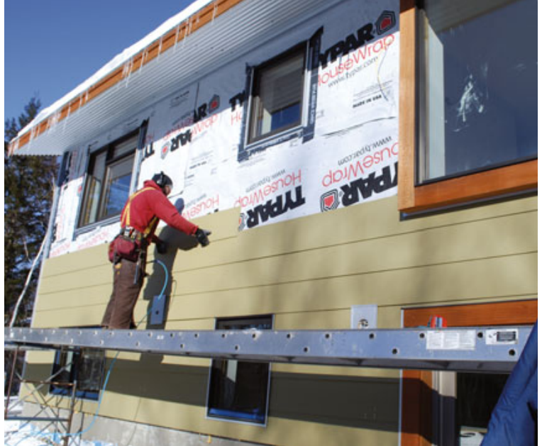
Figure 6. Spray-foam was used to seal the plates and boost R-values at the truss heels, and any open stud bays were filled with damp-spray cellulose (left). After the sheathing was wrapped with housewrap, window and siding installation was typical (above).
