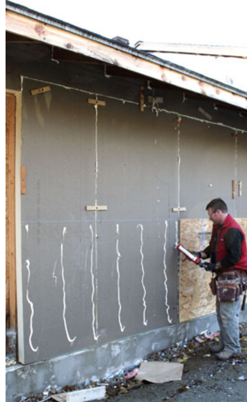
Figure 3. Before installing the AdvanTech sheathing, the carpenters cut slots for biscuit joints in the butt ends of the panels (left) and predrilled countersunk holes for the structural screws (above left). The sheathing was also glued to the foam panels with a low-VOC construction adhesive (above right).
